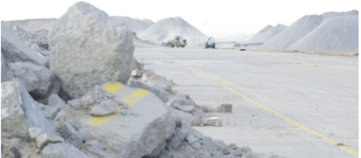
Above: Rubble still showing the runway markings undergoes recycling on North Stapleton. Below left: The terminal demolition underway around the
