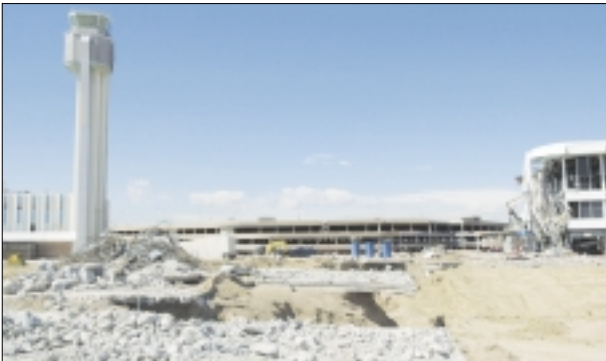
Above: Rubble still showing the runway markings undergoes recycling on North Stapleton. Below left: The terminal demolition underway around the
