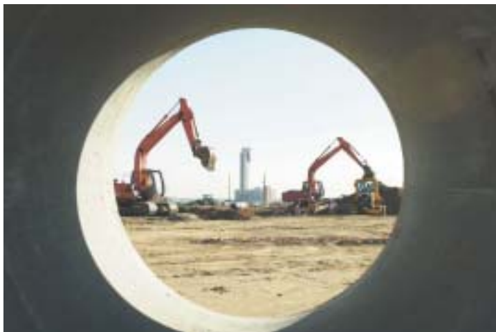
Construction of infrastructure in Stapleton's first neighborhood.
