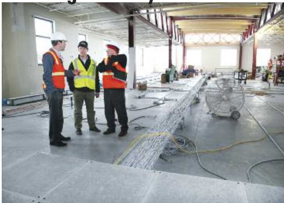
The photo shows the main part of the library looking to the east. The technical, electrical and IT systems are being installed and will ultimately be under the raised flooring.
