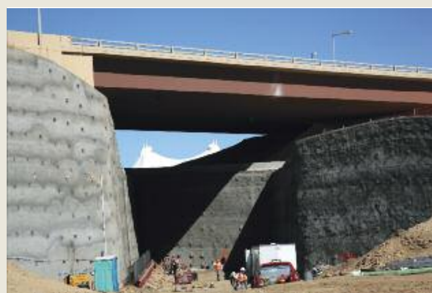
As the RTD commuter rail line reaches DIA, it will pass between the two giant retaining walls that support access roads to the terminal building. The center wall that now blocks the path of the train is necessary during construction and will come down once the bridges are complete.
