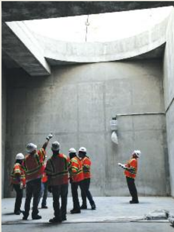
To manage exhaust in the underground Regional Bus Facility, an extensive fan system pulls air from below and blows it out exhaust stacks, shown above.
