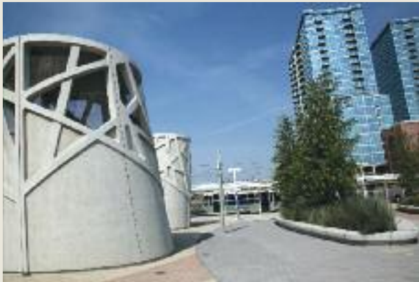
To manage exhaust in the underground Regional Bus Facility, an extensive fan system pulls air from below and blows it out exhaust stacks, shown above.
