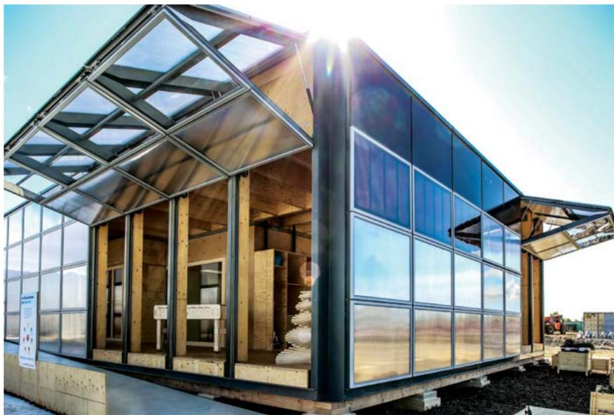
Above and right: the Swiss team's NeighborHub structure will return to Fribourg where it will become a co-working space attached to the blueFACTORY, a research and development center for the built environment of the future. The walls are all "productive" supporting solar panels, plants, aquaponics and solar dryers. A "dry" toilet
