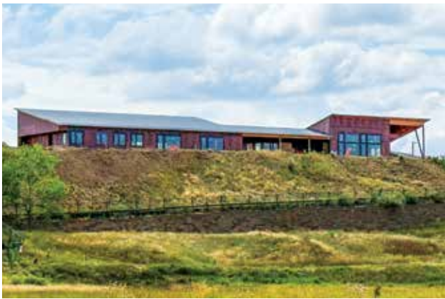
The new building at Bluff Lake Nature Center.
